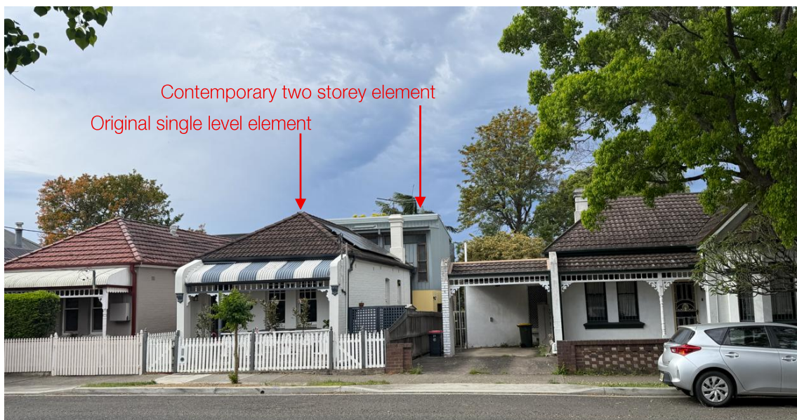
Figure 2: Subject site, viewed from the street frontage
