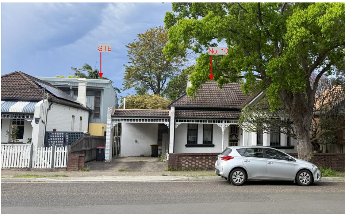
Figure 7: No. 10 Hampden Street as viewed from the street frontage
